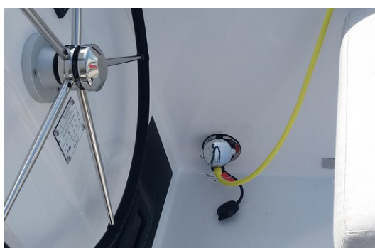
Shore power socket in starboard helm
